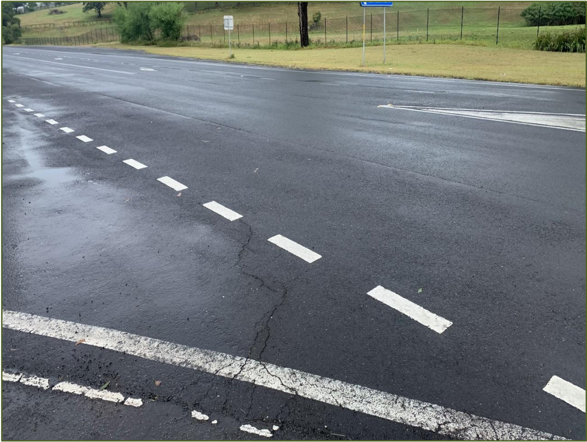
Figure 2.0.8 – Meandering Cracking
