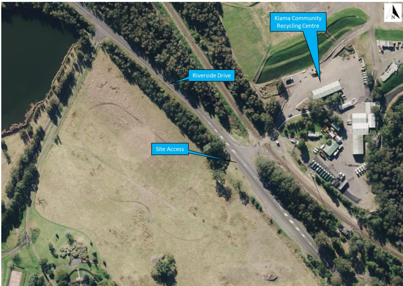
Plate 4.1 Site access from Riverside Drive
