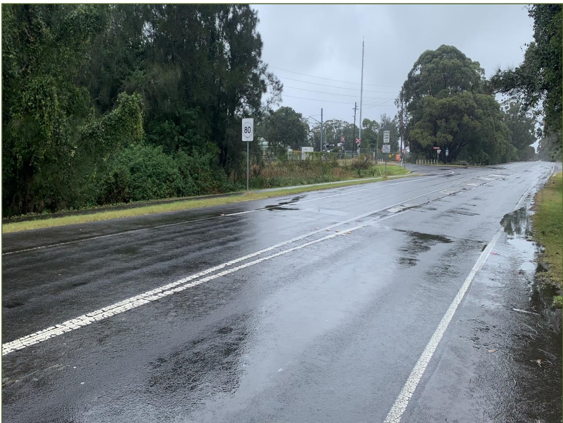
Figure 2.0.7 – Minor Rutting
