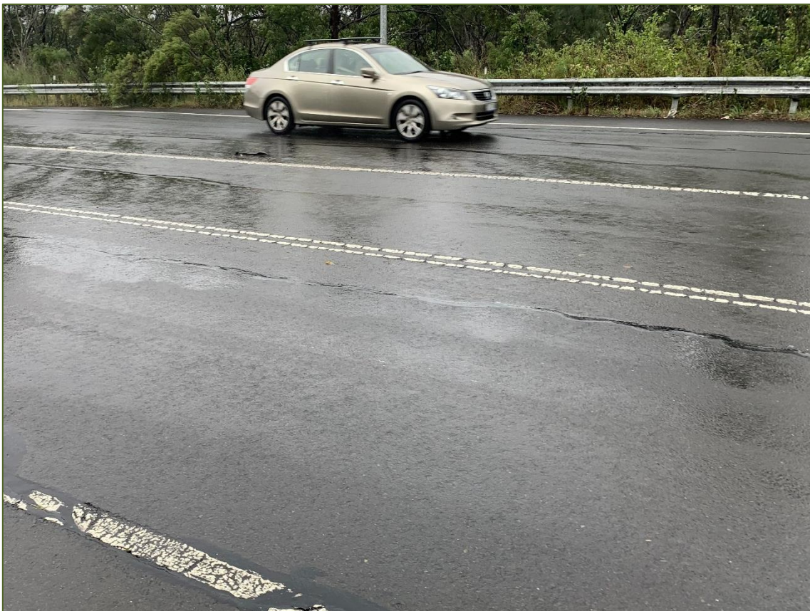
Figure 2.0.3 – Slight Rutting
