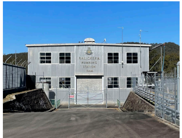
Balickera Pumping Station
