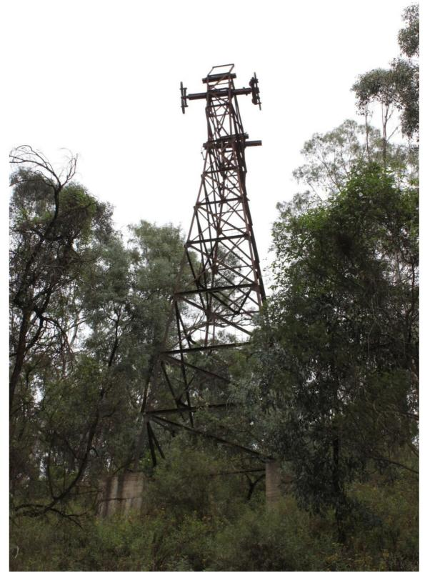
Tower 1 (MS04\_2) is an example of a complete pulley tower. This tower is directly opposite the lime kiln group (refer to Figures 3.1 and 5.1 and is the only surviving complete and standing tower (IMG\_9030).
