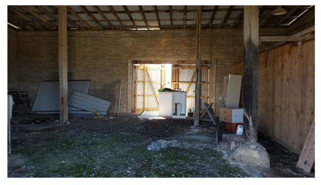
Plate 3.13 Interior of control room showing wooden beams for piles and roof, concrete foundations and dirt floor (20151006\_144957).
