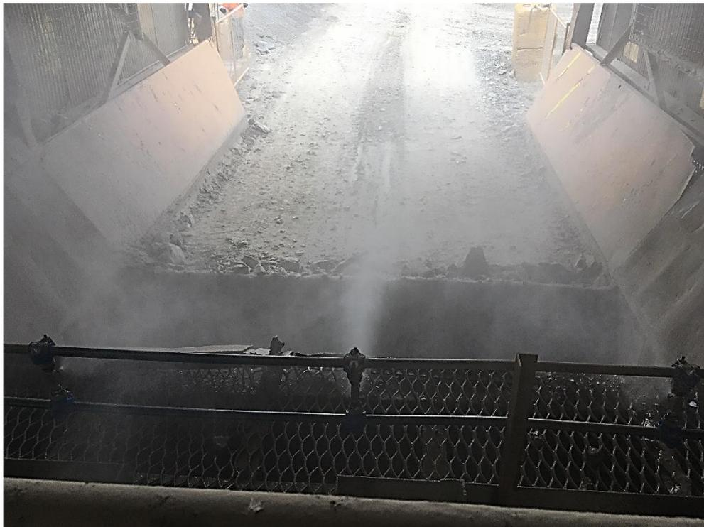
*Fogging system installed in the Primary crusher tip chute*
