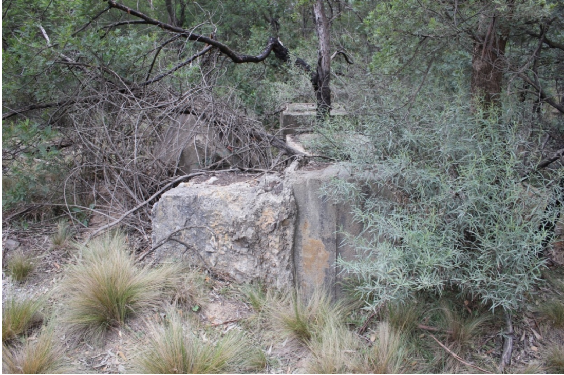
Plate 3.8 Example of an upturned concrete plinth showing both above and below ground sections (IMG_8992).
