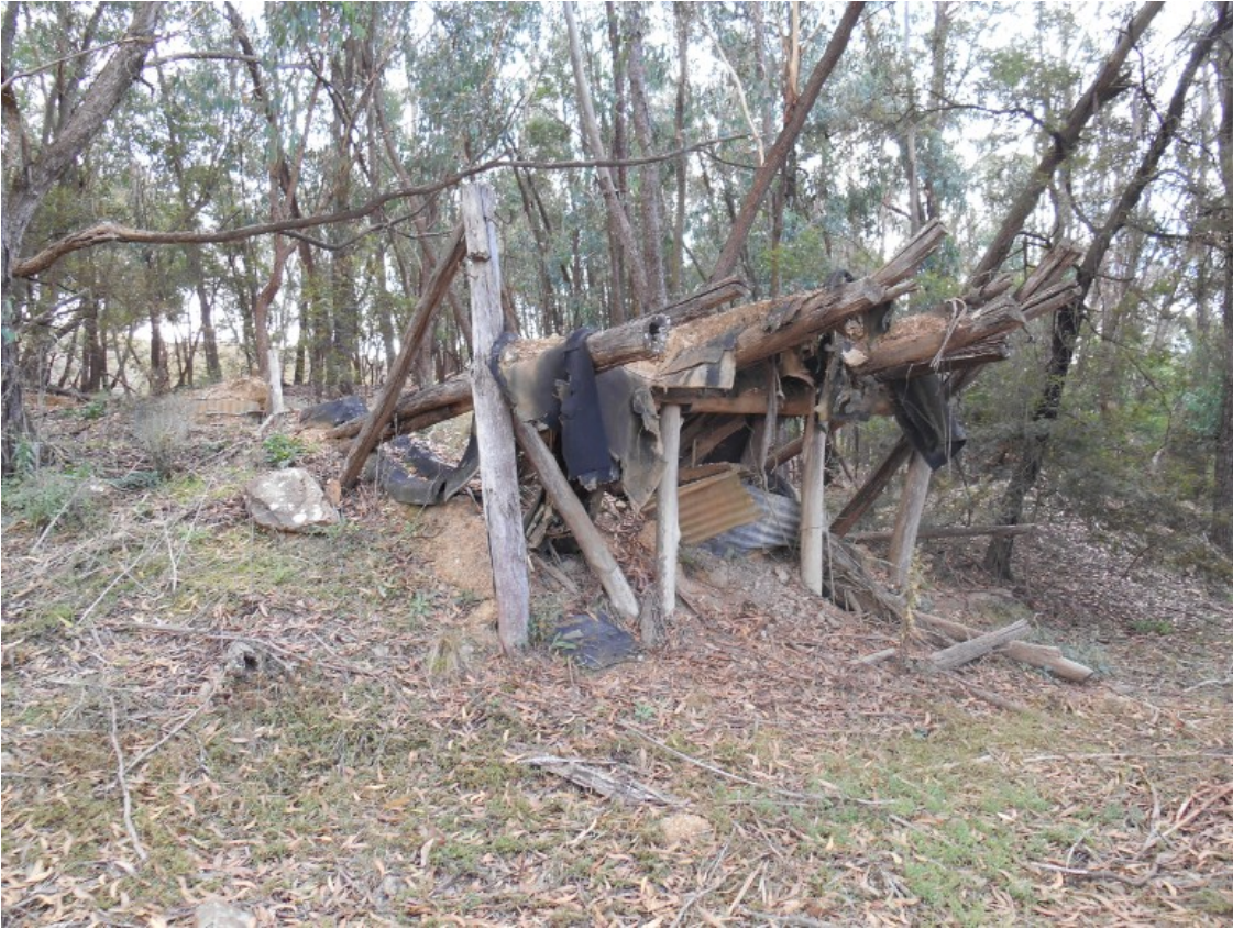
Plate 3.37 MS11 loading ramp (DSCN1067). View north-west.
