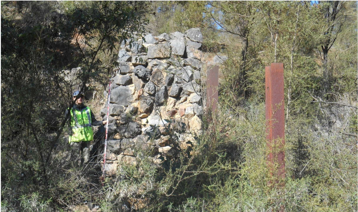
Plate 3.1 Kiln Area A showing one remnant kiln and associated iron beams (DSCN2491).
