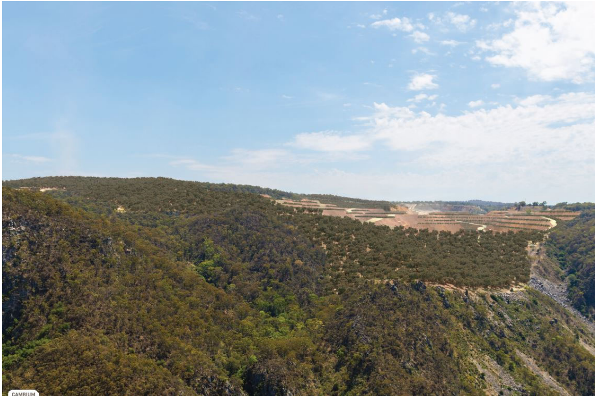
Plate 3.41 Photomontage of the view to the mine pit from the Bungonia Lookdown 5 years after the end of the proposed 30 years of continued mining operations. (Source: RLA 2018 and Cambium).
