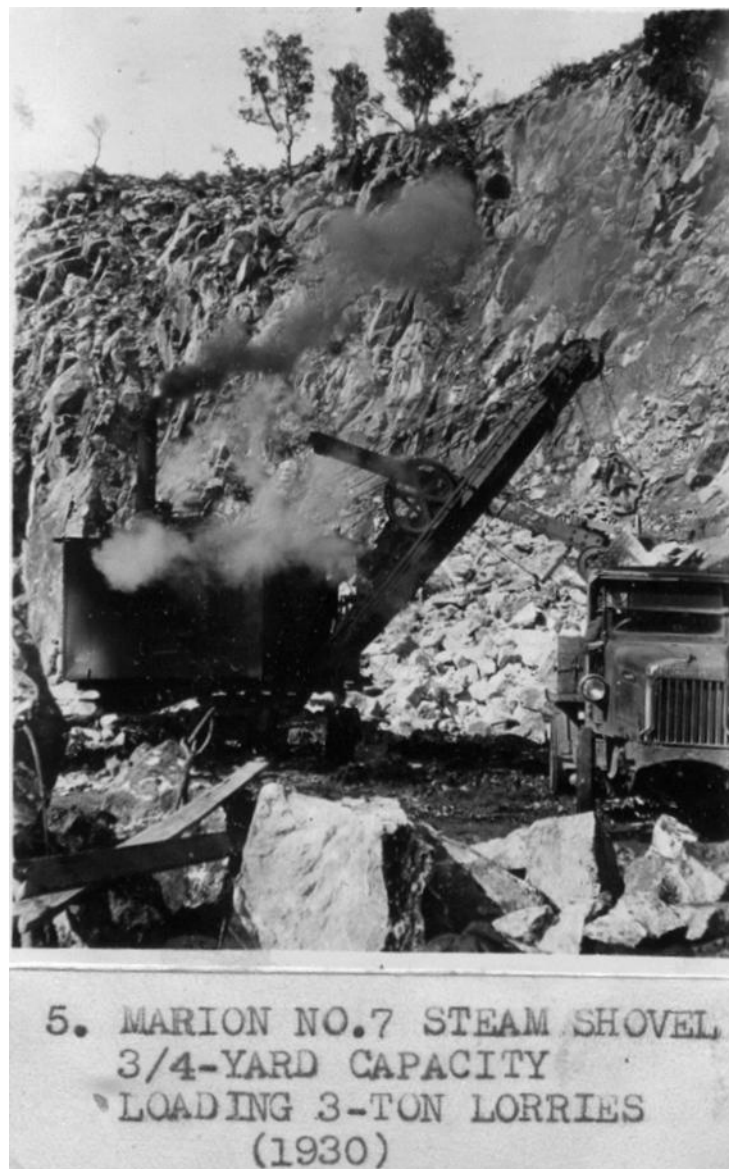
Plate 2.14 An example of the steam shovel and lorries used in the mine in the 1930s (Boral Cement Limited 2015).
