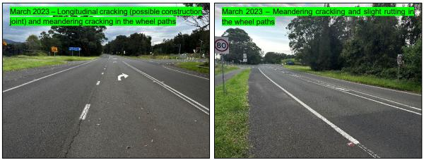
Figure 2.0.3 – Pavement Defects Encountered During the visual inspection on 26<sup>th</sup> March 2023
