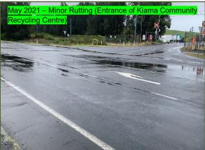
Figure 2.0.2 - Pavement Defects Encountered During the visual inspection on 6th May 2021
