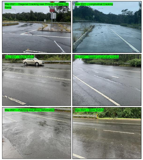
Figure 2.0.1 – Pavement Defects Encountered During the visual inspection on 6th May 2021
