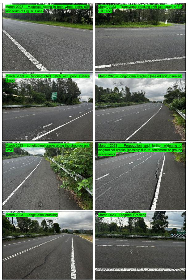
Figure 2.0.4 – Pavement Defects Encountered During the visual inspection on 26th March 2023
