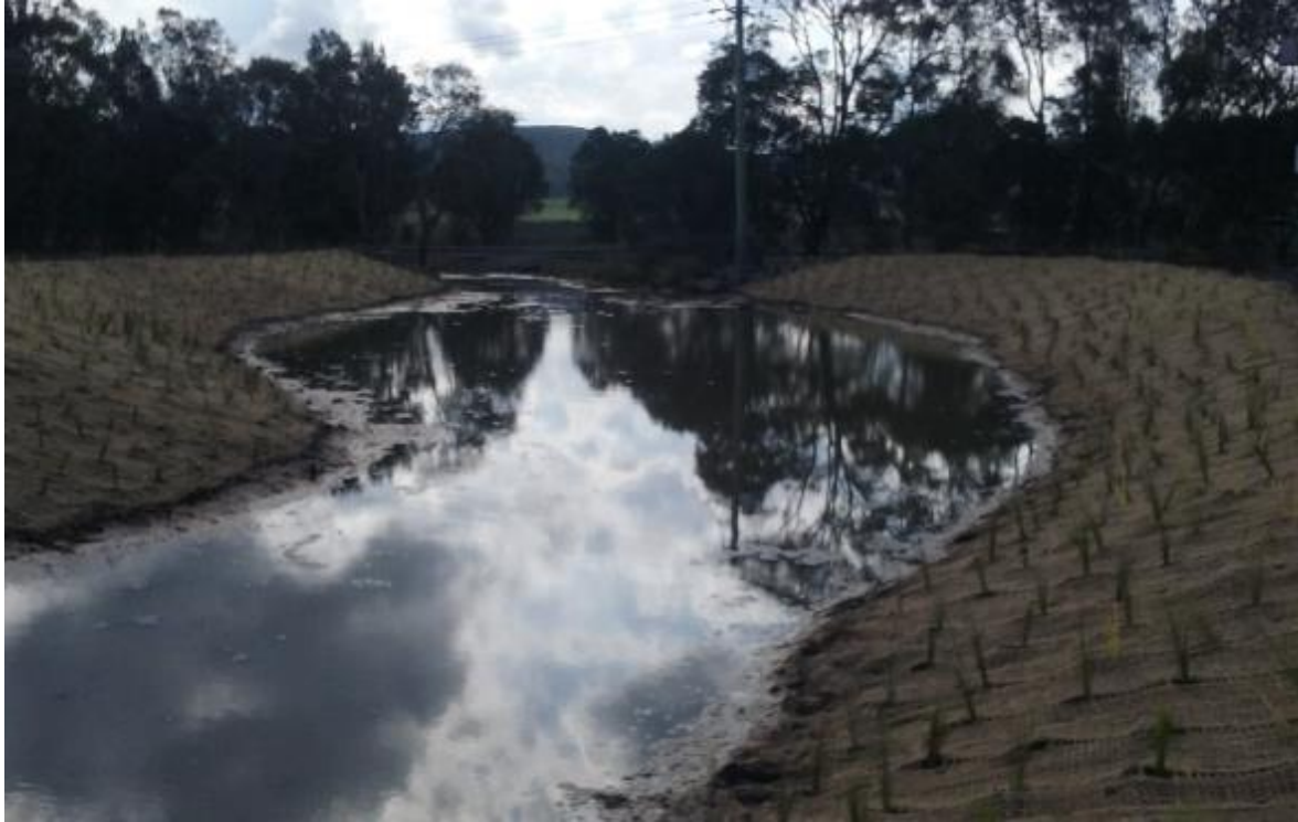
FY17 Re-aligned Western Tributary Rehabilitation Progress
