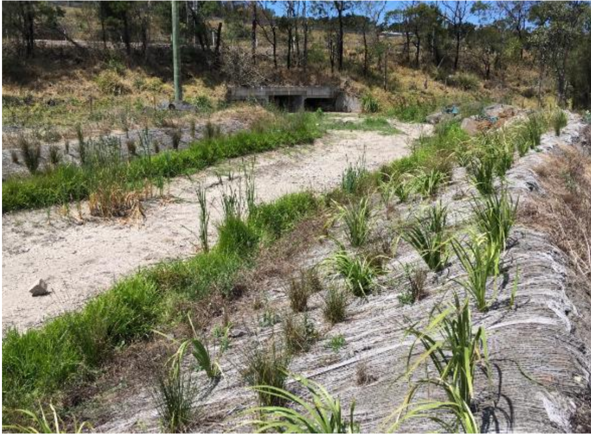
FY18 Re-aligned Western Tributary Rehabilitation Progress
