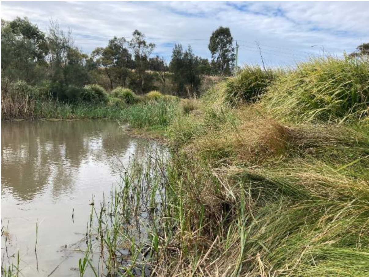
FY22 Re-aligned Western Tributary Rehabilitation Progress
