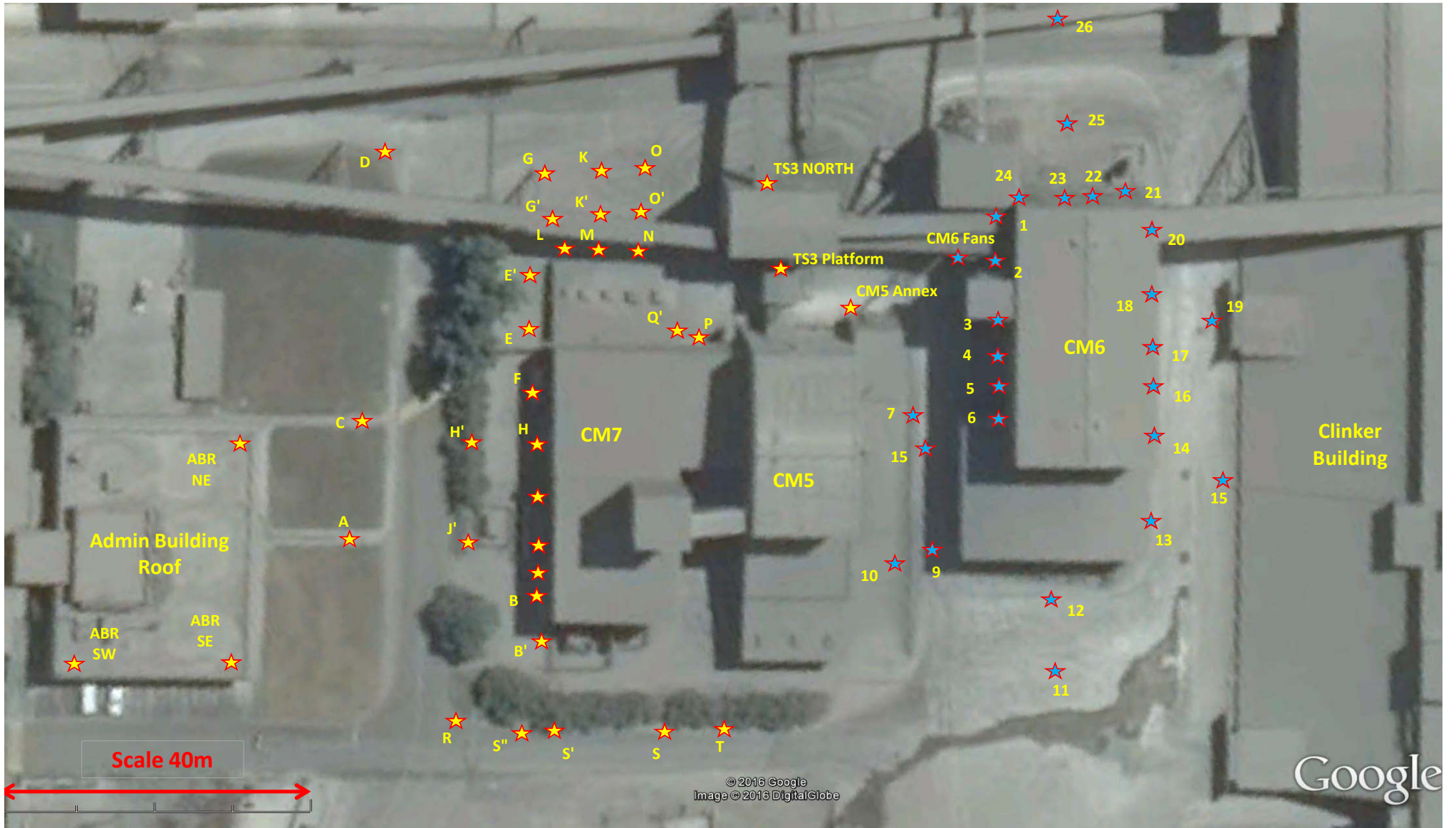
Figure 3.7A: Aerial view of Cement Mills 6 and 7 and measurement locations
