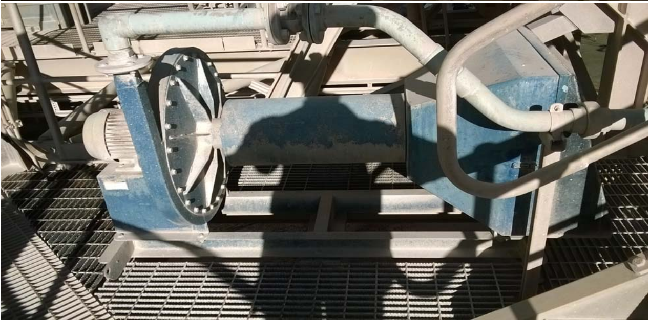
Figure 3.6: Area on top of the Raw Meal Silo Building near FA260 where noise from the baghouse fan below causes elevated sound levels
