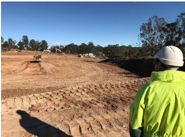
Large scale earthworks have resulted in an estimated **18000 tonnes** of earth being moved, creating the 'floor' that the new plant will eventually sit upon.
