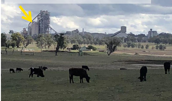
SWDF 'tube' conveyor and equipment
