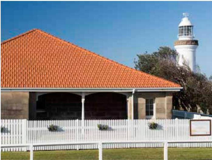
However, up until recently, the buildings surrounding the lighthouse weren't in great shape. "The roof tiles were rapidly deteriorating and water was entering the roof space, which was causing damage to the historic fabric of the building," Ms Stubbings recalls. As a result, the Norah Head Lighthouse Reserve Trust enlisted the help of LMR Roofing to reroof the buildings using Boral's French™ profile terracotta tiles in Sydney Red.
