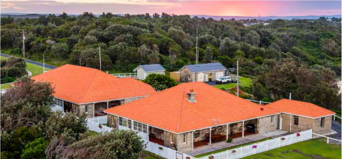
“The contractor only had three weeks to reroof the buildings, with extras including heavy duty sarking, canter battens, barge and ridge and insulation batts, but they managed to meet the tight deadline and worked in a most efficient, professional manner,” commented Ms Stubbings.
