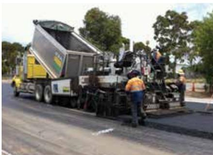
WarmPave asphalt with 15% RAP being paved on the Superway project in South Australia.
