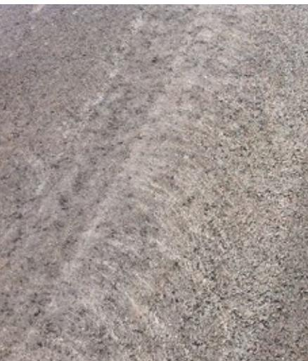
Typical scuffing caused by the rubber tyres of forklifts and reach stackers when handling fully laden containers.
