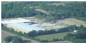
Brick plant under construction, Terre Haute, Indiana
