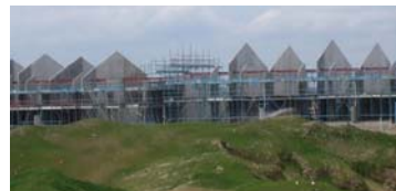
Grotto Precast townhouse development, NSW
