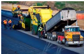
Construction of EastLink, Melbourne
