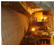
Berrima cement mill 7 upgrade
