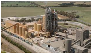
Waurn Ponds cement works
