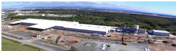
Plasterboard plant under construction, Pinkenba, Queensland
