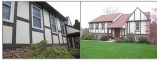
Repair & Remodel – Lancaster, PA
