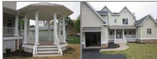
Single Family New Construction – Middle River, MD
