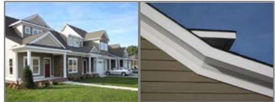
Multi Family New Construction – Gloucester, VA
