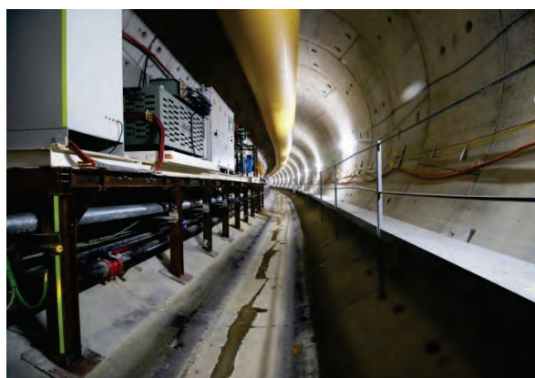
Forrestfield Airport Link, WA (Photo supplied courtesy of Salini)
