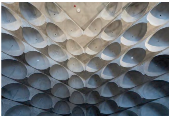
Boral supplying Envisia concrete to Crown Sydney Barangaroo, NSW
