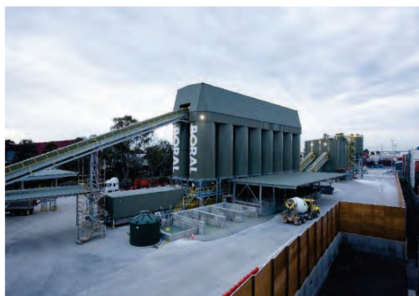
New West Melbourne Concrete Plant, Vic
