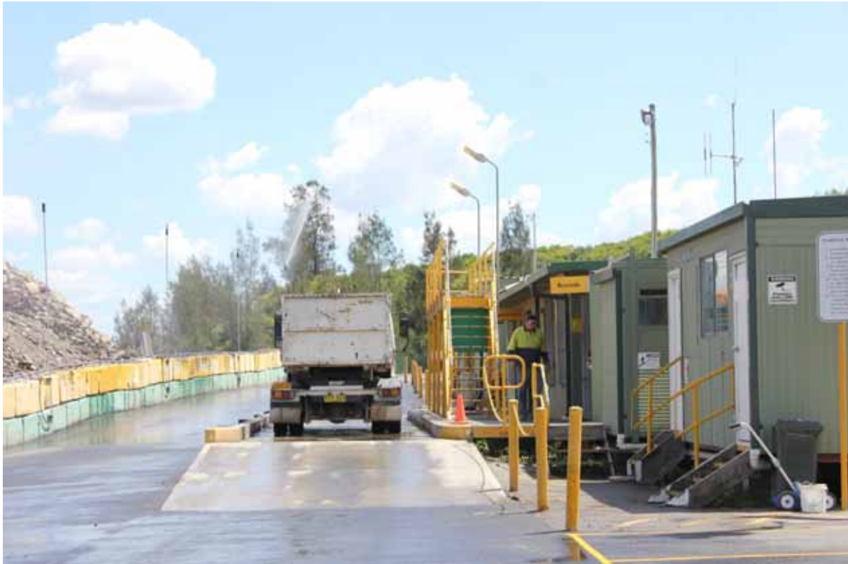
Photograph 2.1 Receivals area, weighbridge and site office
