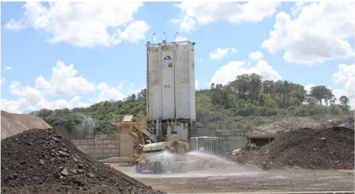
Photograph 14.4 Photograph taken within the site showing stabilisation processing plant, looking north towards vegetated ridgeline immediately north of the facility which provides visual screening
