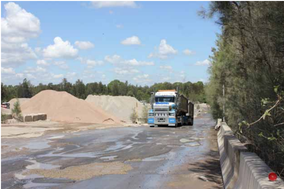
Photograph 2.5 Perimeter haul road
