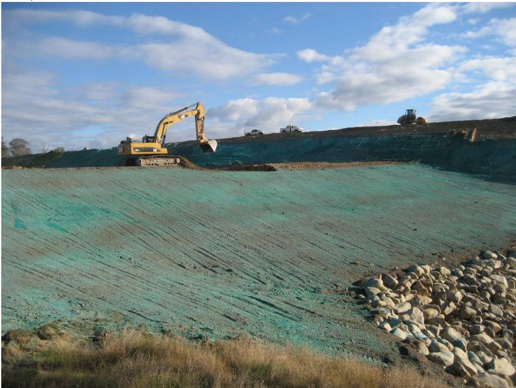
**Plate 15 - Hydromulching of Completed Batter Slopes**
