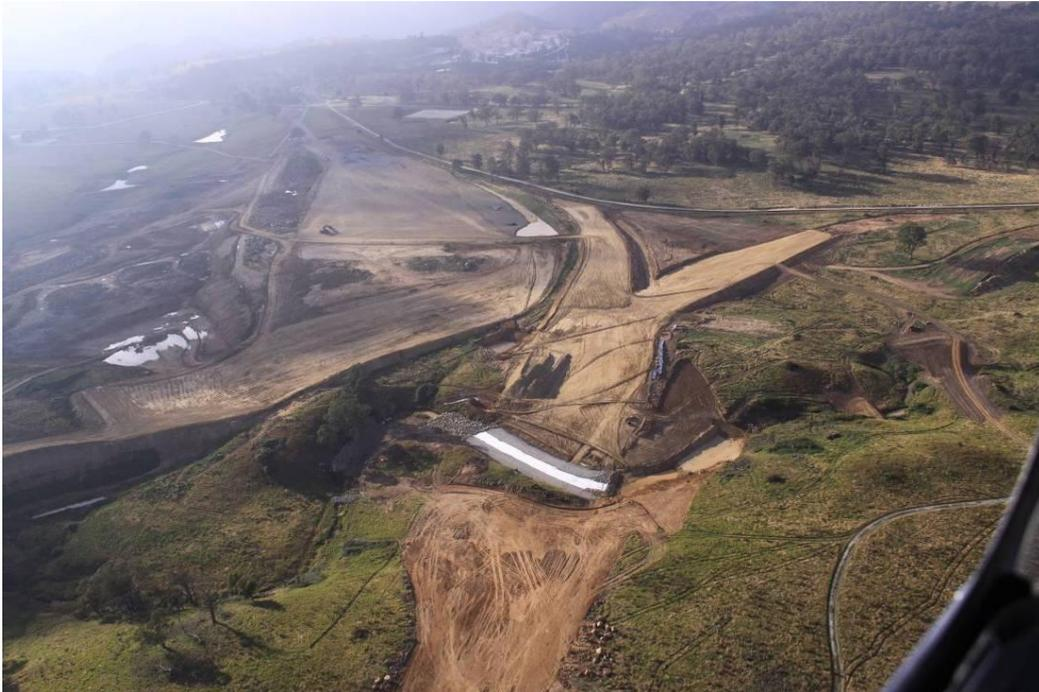
**Plate 8 - Drainage Blanket During Construction**
