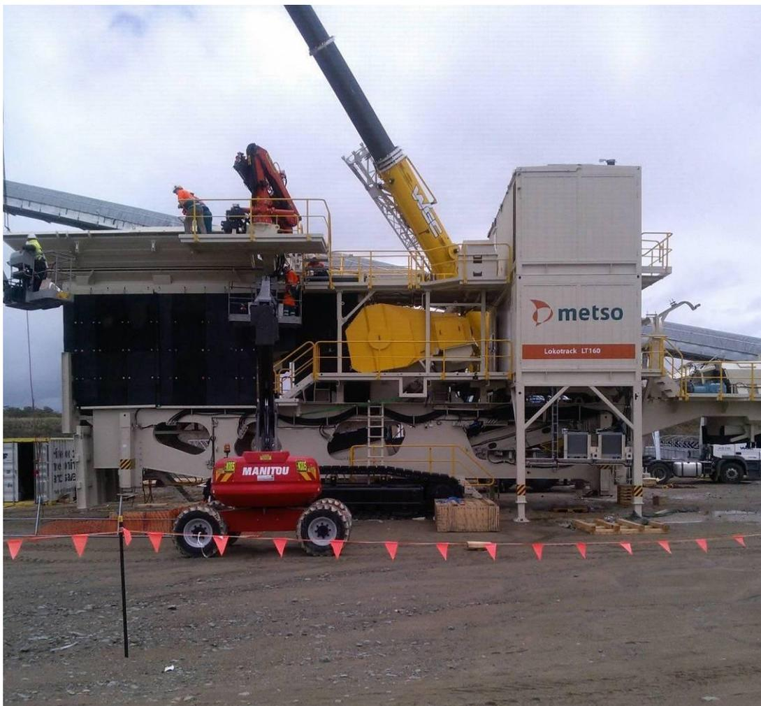
**Plate 2 - In-Pit Crusher under construction**
