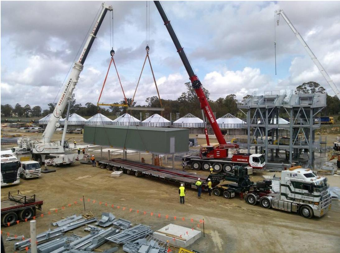
**Plate 3 - Construction of Processing and Material Handling Infrastructure**
