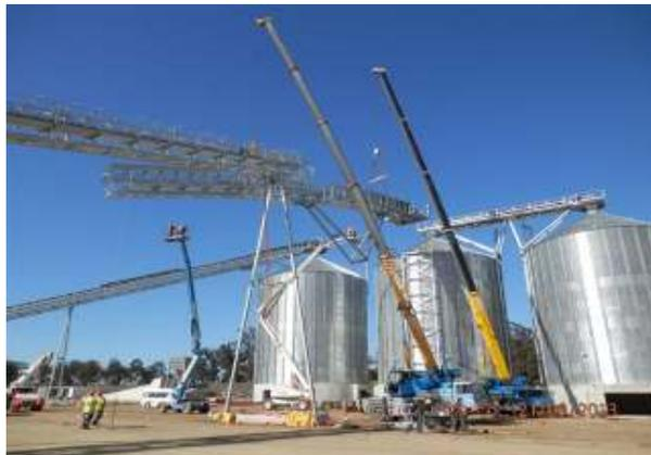
*Lifting the conveyors in place*
