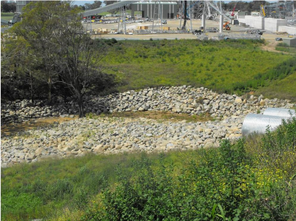
**Plate 11 - Rock Protection in Tangarang Creek Downstream of the Railway Embankment**
