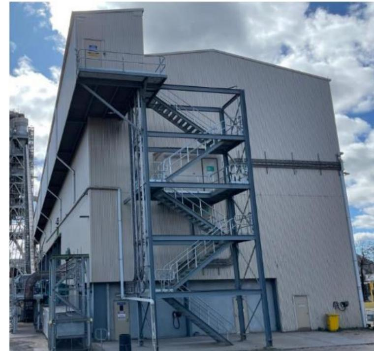
Figure 22 - Site photo showing external steel stair at south end of nearest building
