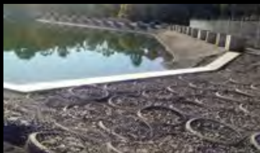
Part of the stormwater management system at Ormeau Quarry
