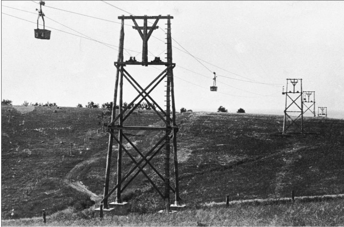
The four mile rope-way communication between the Brighton Cement Works and Reynella Quarry (1920)
