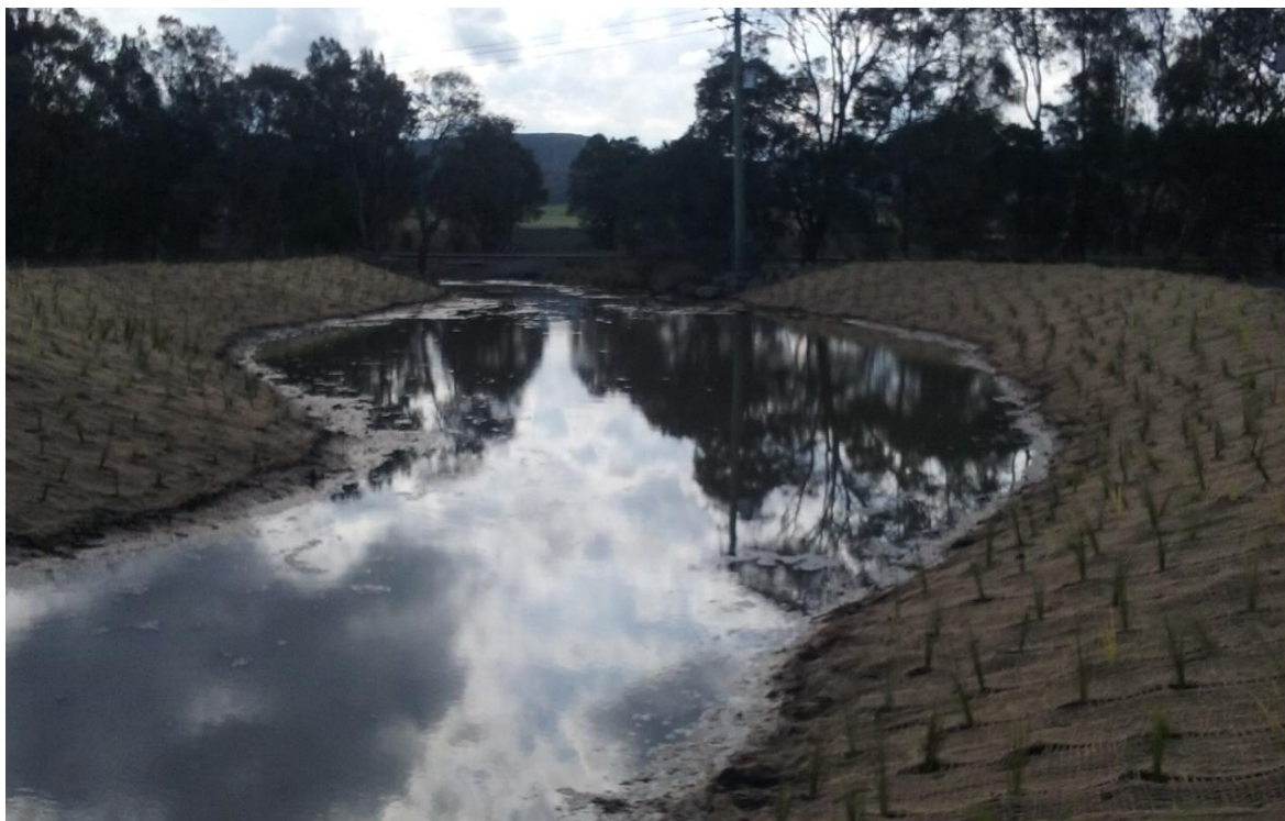
FY17 Re-aligned Western Tributary Rehabilitation Progress
