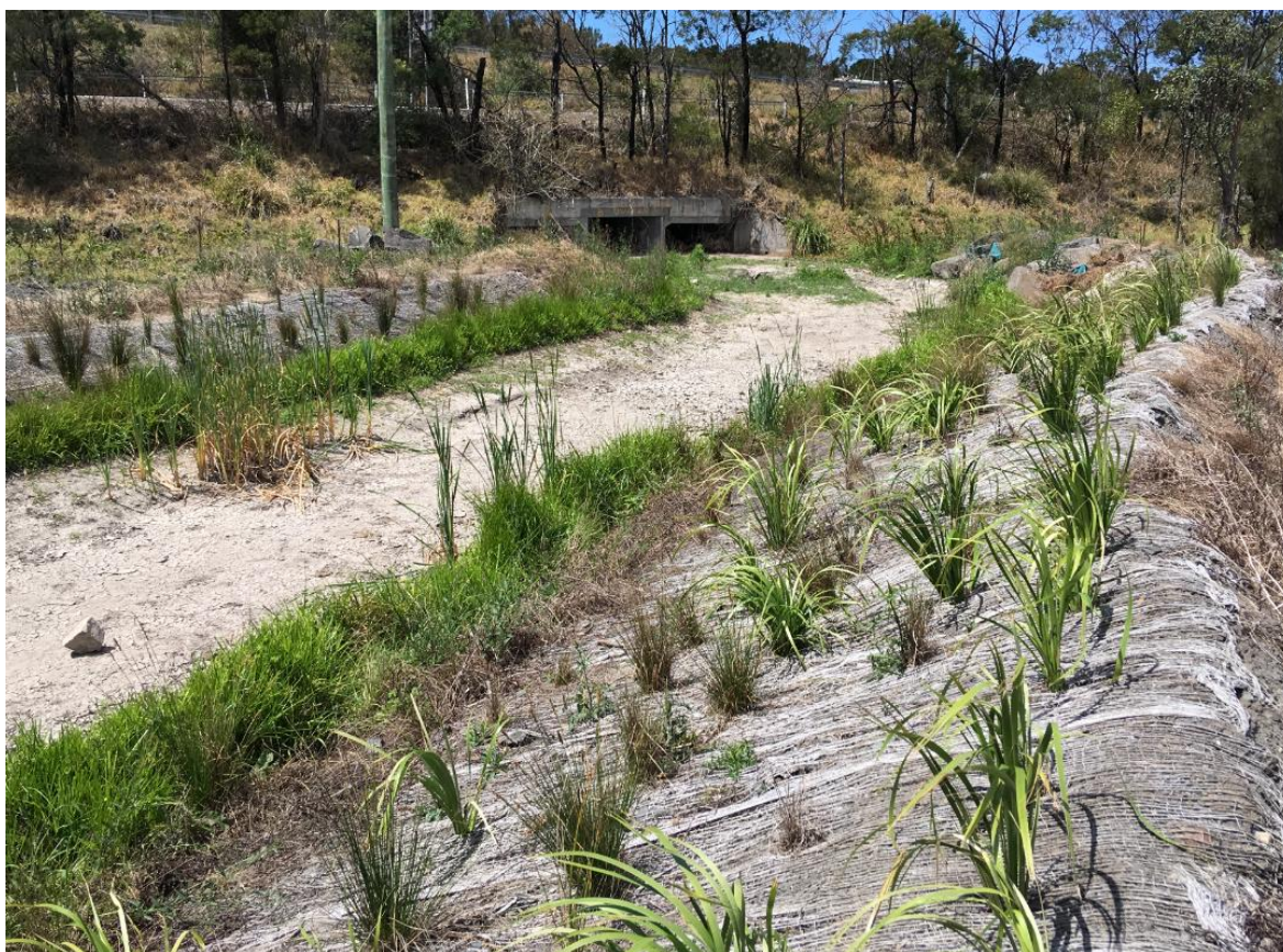
FY18 Re-aligned Western Tributary Rehabilitation Progress
