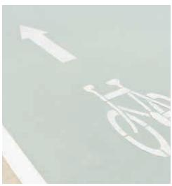
The **colori**® range includes a choice of coloured concrete options which then incorporate various textures, lines, patterns, shapes and other effects into the concrete surface to create an innovative finish. **colori**® concrete oxides colour the full depth of the entire mix not just the surface to provide a rich colour.
