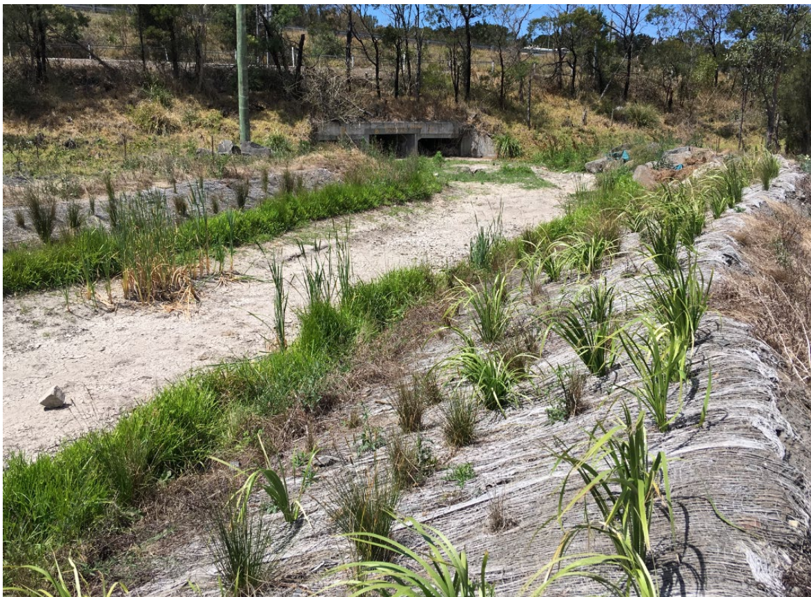
FY18 Re-aligned Western Tributary Rehabilitation Progress
