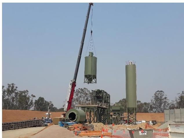
A crew of **six** supervised the installation of the silos and other elements requiring a crane lift, including the plant's **materials conveyors**.
