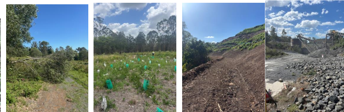
Chainsaw fallen tree, Back pack spray reveg, seed spreading drain ,backpack spray workshop/control room area
