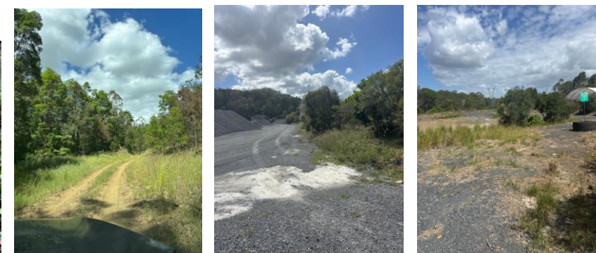
HV spray offset tracks, HV spray blending plant walls and sediment C basin
