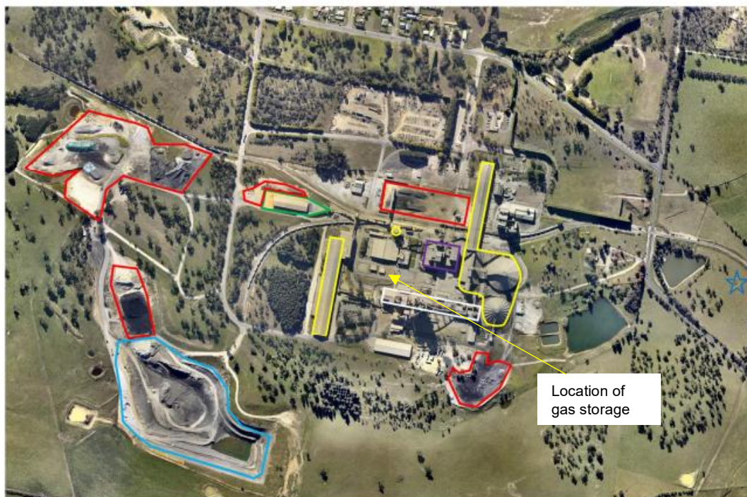
Figure 13 Location of Gas Escape Incident
