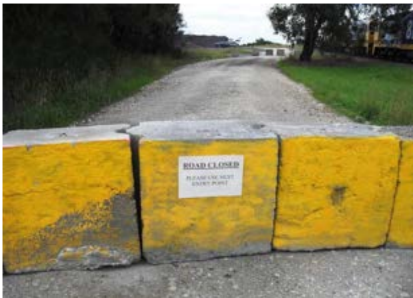
Photo 3: Rock blocks in place to restrict vehicle movements to the stockpile area.
