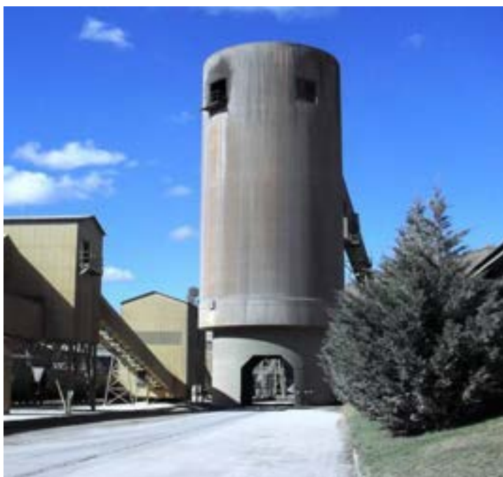
Photo 4: Silo for the loading of clinker into trains and trucks
