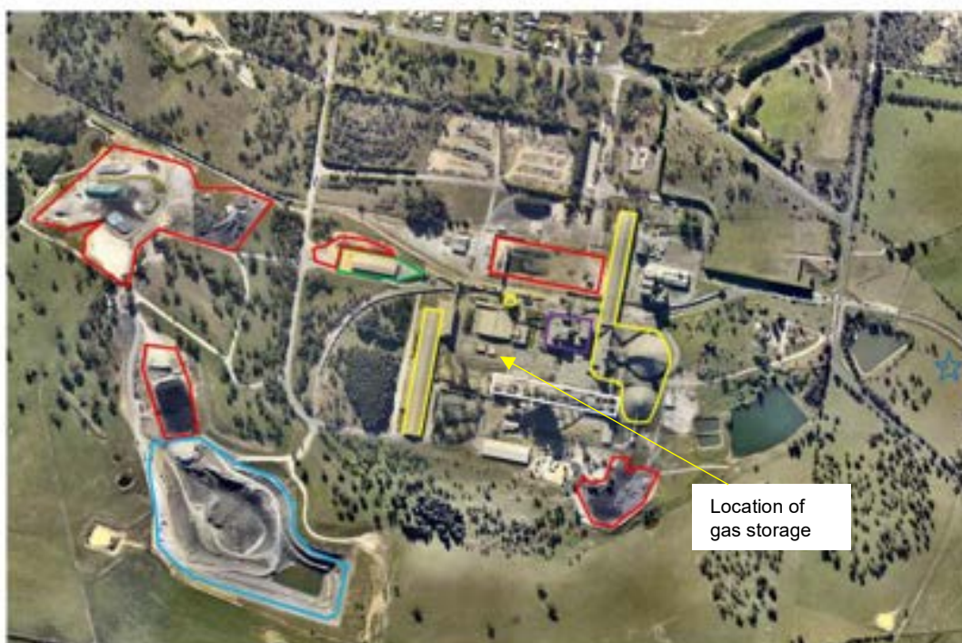
Figure 13 Location of Gas Escape Incident
