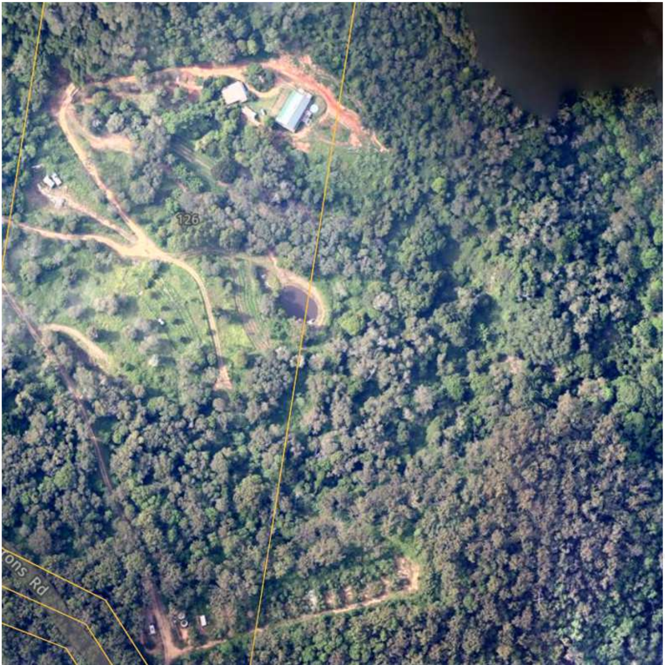
Figure 5: Aerial showing the western boundary of the offsets site and the prior encroachment into the site unknowingly by neighbouring landholders.
