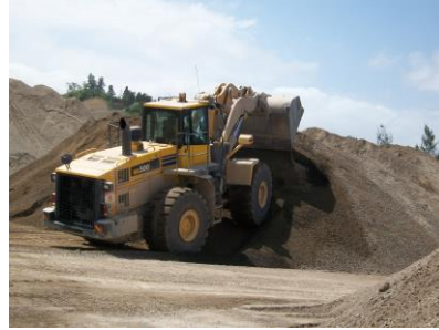
Step 8 - Inspection Point 3 (Waste Storage Area – Finished product)
