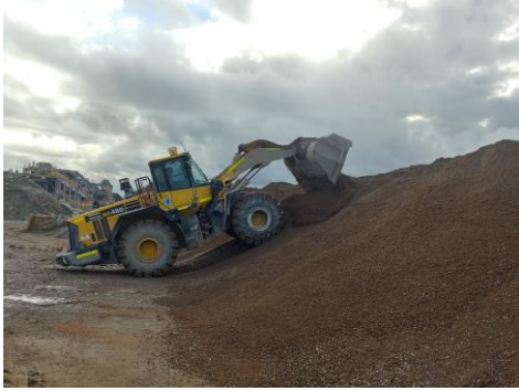
Step 7 - Inspection Point 3 (Waste Storage Area – Finished product)
