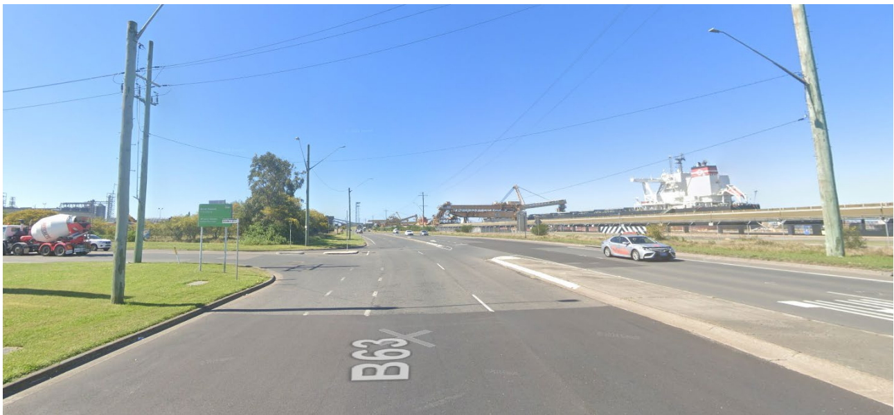
Plate 3.1 Cormorant Road (looking east towards Egret Street)
