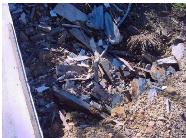
Photo 7 – Flat Asbestos Cement sheet fragments
