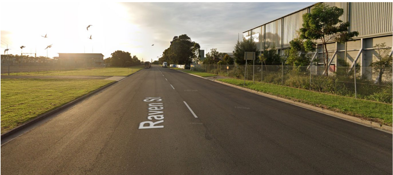
Plate 3.3 Raven Street (looking east)
