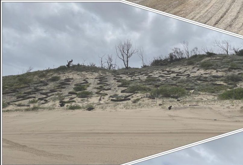
Plate 3: View south taken from the Haul Road on the southern end of Pit 7 showing coir logs in rehab area (Ref: E822M_0076)
