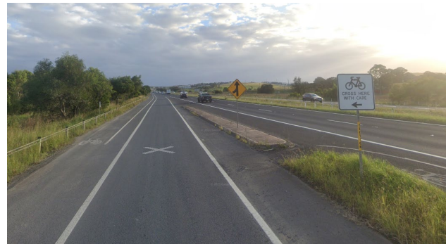
Cyclist crossing at northbound on-ramp to Princes Highway
