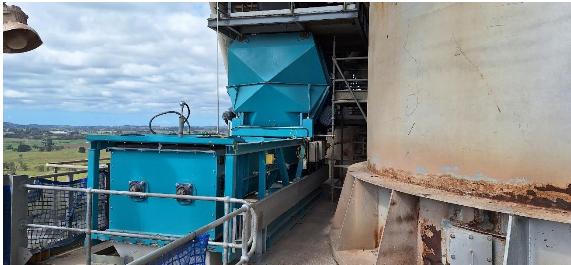
Plate 4 – Multiflex System which Weighs SWDF Fed into the Plant
