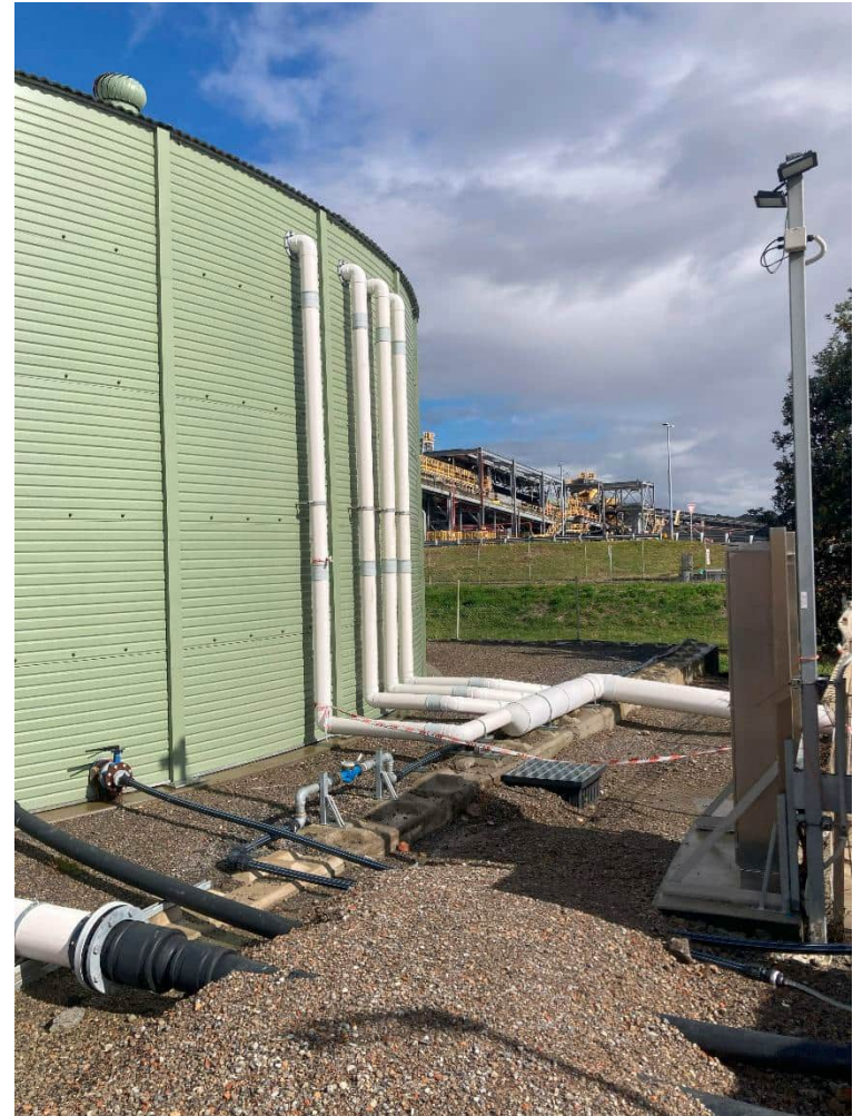
Photo 6: Tank Storage and Pipework (19 August 2025)
