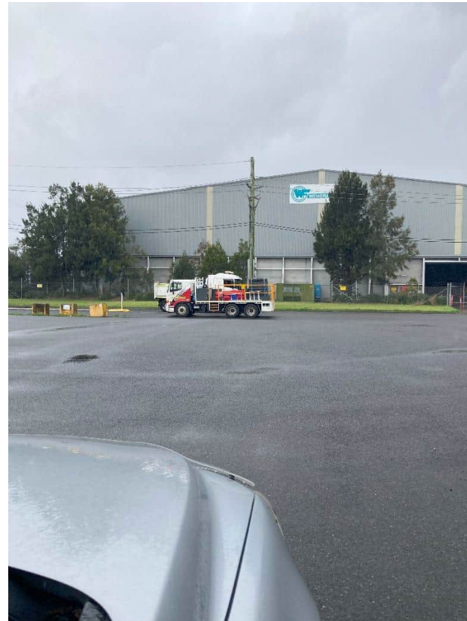
Photo 22: Site Entrance – No Mud Tracking (19 August 2025)
