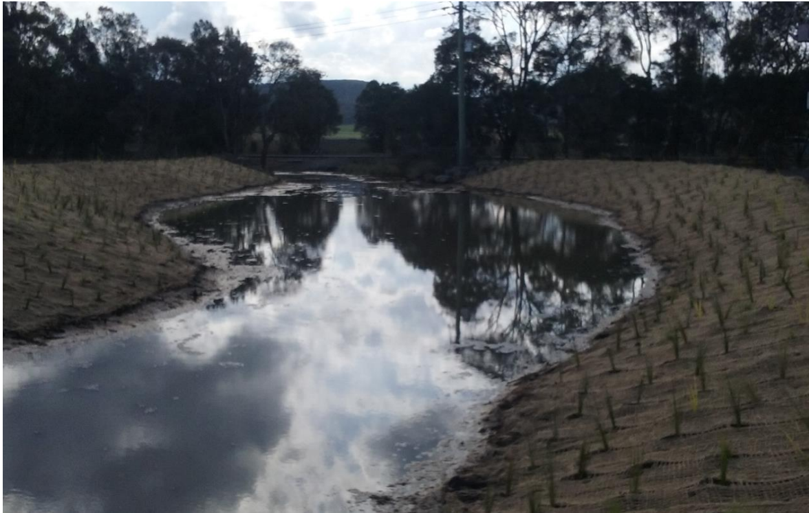
FY17 Re-aligned Western Tributary Rehabilitation Progress
