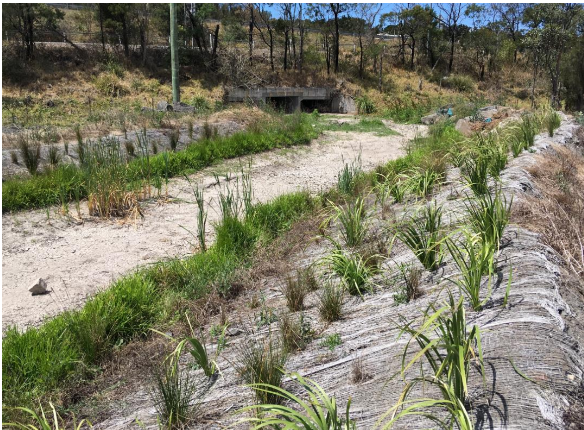
FY18 Re-aligned Western Tributary Rehabilitation Progress
