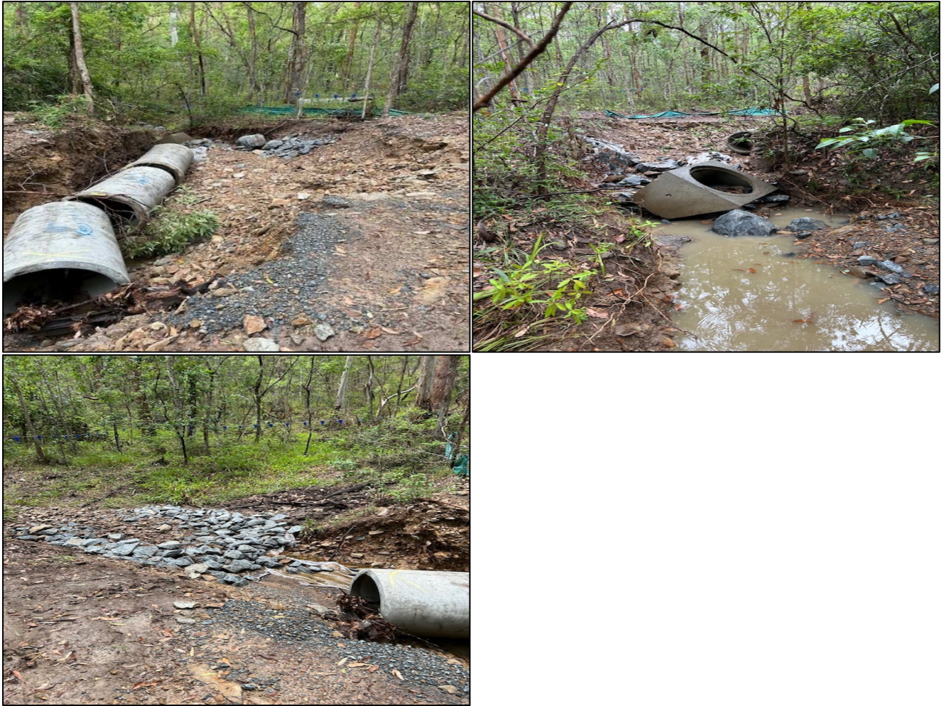
Photo set 4: Damage to crossing, dated 8 January 2024.
