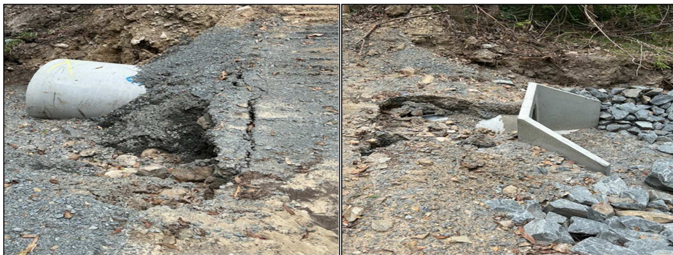
Photo set 3: Washout at Headwall, photos dated 19 December 2023.
