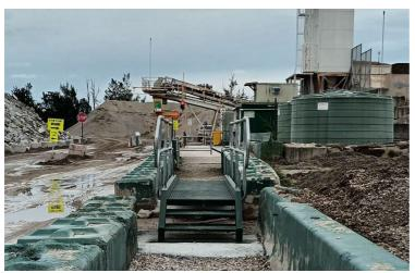
Figure 5. Repaired walkway over internal drain
