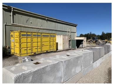
Figure 4 – Self-bunded enclosed chemical storage
