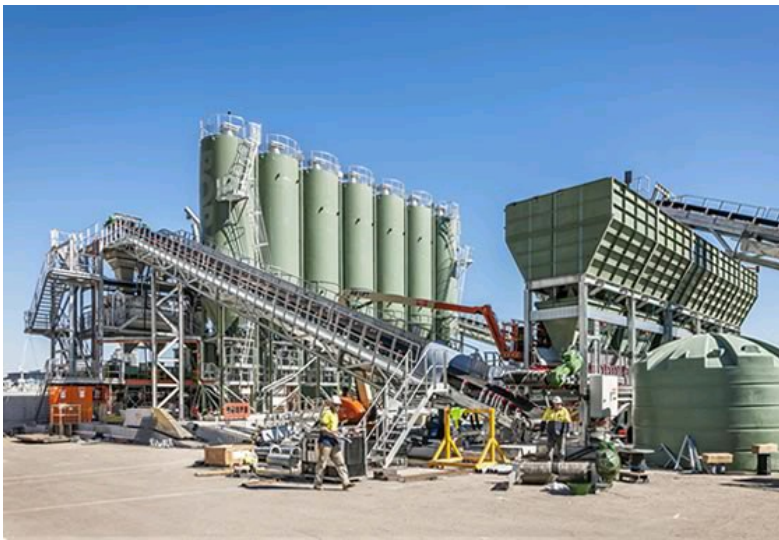
Boral's Onsite batch plant
