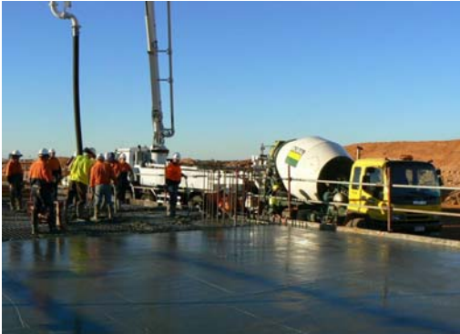
Foundation for the Secondary Crusher at Boddington Gold Mine
