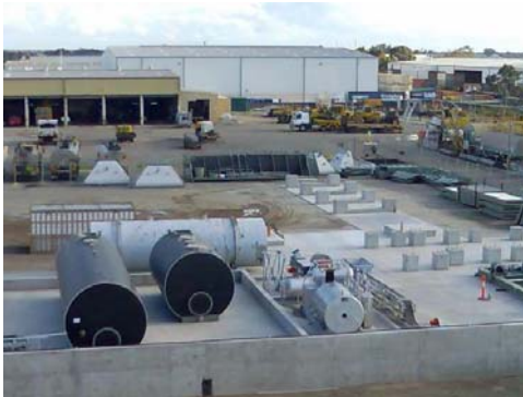
Foundation for the new asphalt plant at Welshpool, WA
