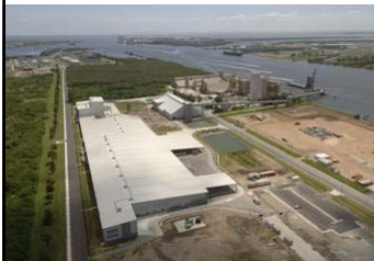
Pinkenba Plasterboard Plant
