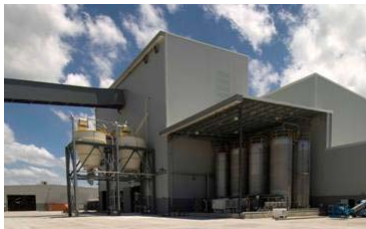
Loading station for bulk plaster trucks
