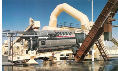
High capacity mobile asphalt plant operating on the Ipswich motorway
