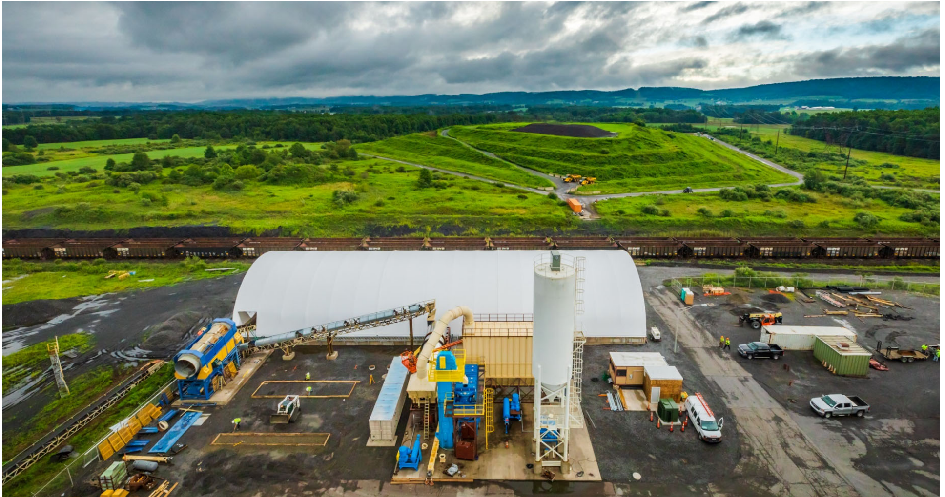
Boral North America's landfill reclaim operation at Montour, Pennsylvania
